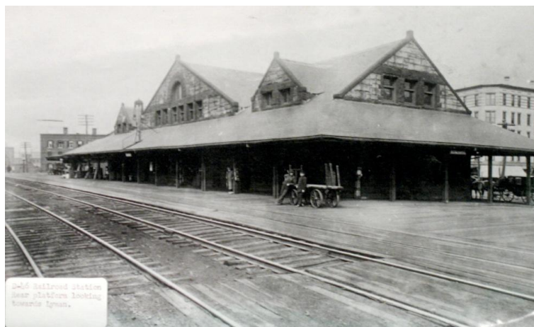
Figure 27: Holyoke Train Station, circa 1885 (photographer unknown), Property of the Archives of the Holyoke History Room of the Holyoke Public Library
