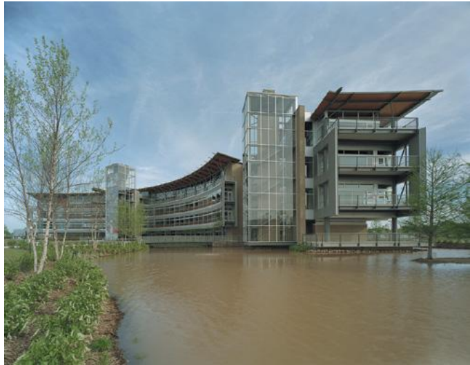
Figure 12: Heifer International Headquarters, Little Rock, AK, continuingeducation.construction.com/article.php?L=5&C=421&P=3
